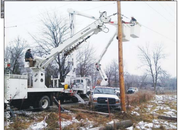
CHEC Linemen replacing poles in Sequoyah County
