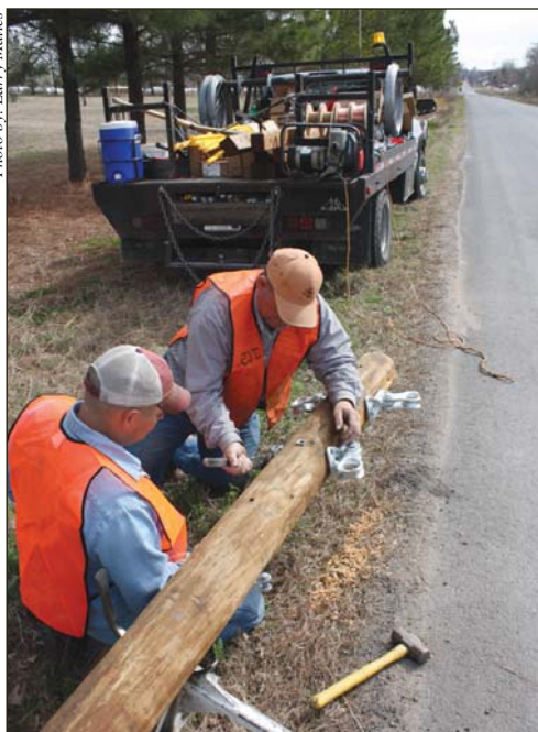
Gordon Construction contractors working on City Lake Road in Stigler.
