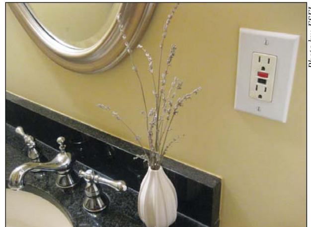
Ground fault circuit interrupter (GFCI) outlets are required in areas around water, near a kitchen or bathroom sink or outdoors, but many older homes do not have these safety measures installed.
